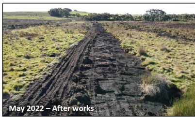
May 2022 – After works
